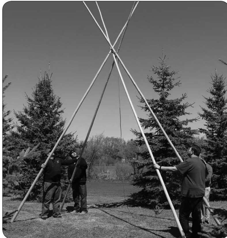
The builders try to form a diamond on what will be the back of the teepee by adjusting the angle of the poles.
